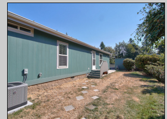
Side Yard View
