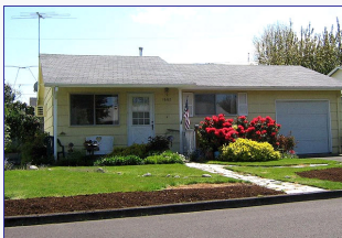
Front Exterior View
